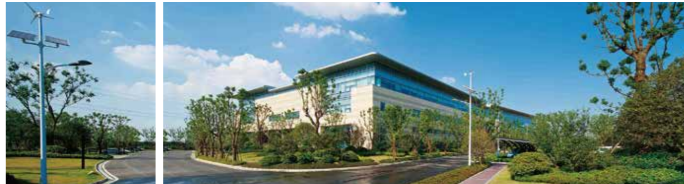
国内首个“六位一体”微能源网 项目：苏州协鑫能源中心 The First “Six-in-One” Micro Energy Network in China: Suzhou GCL Energy Center
